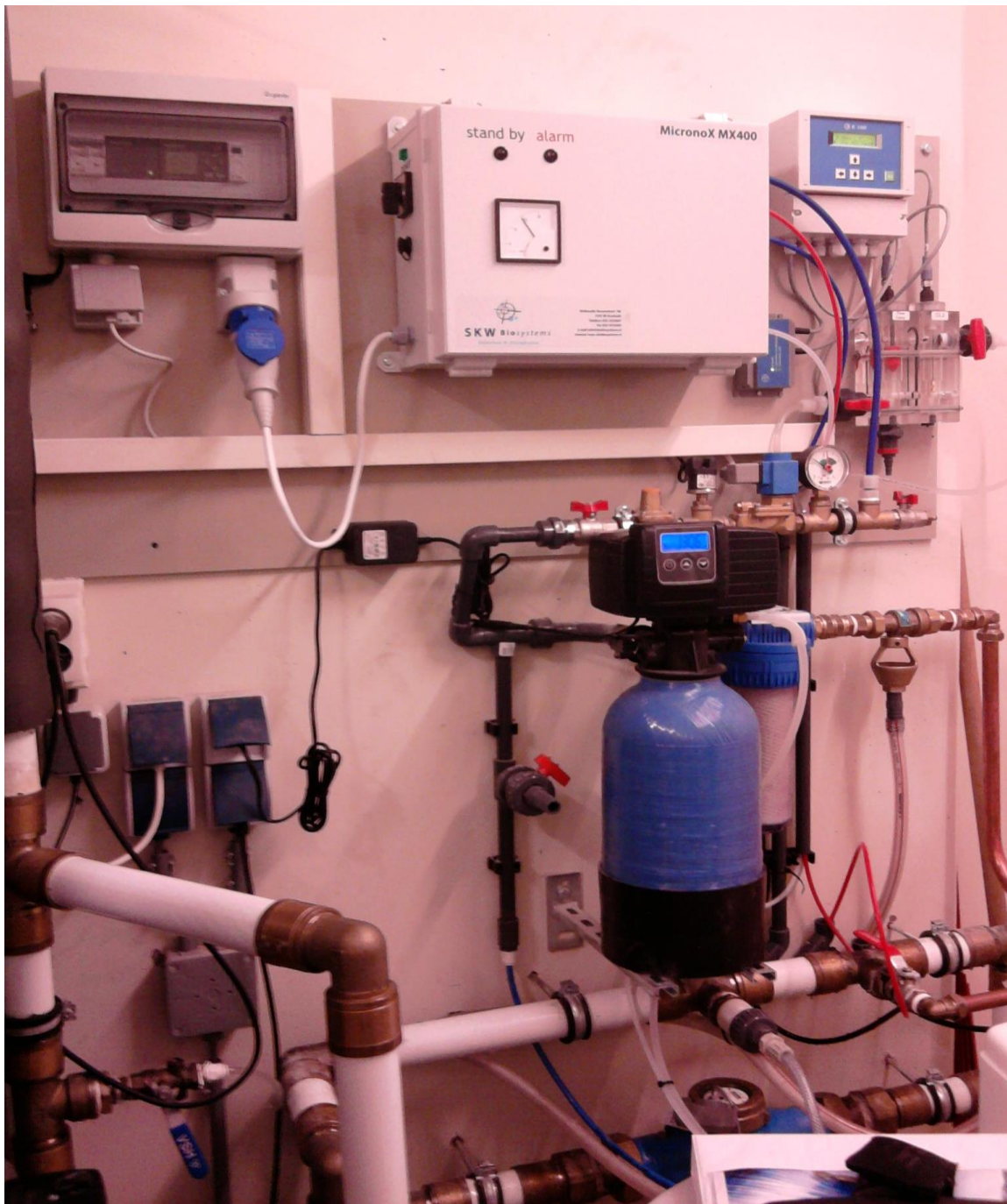
EL 400 with water softener and FAC dosing control
