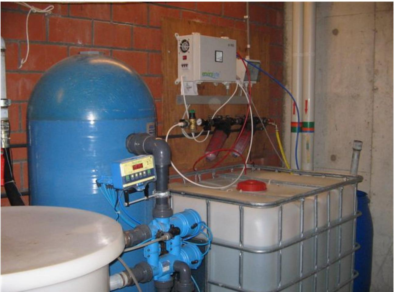
The complete water system is equipped with a water softener. Redox control probe is installed in the water pipe 3 meter after the injection point.
